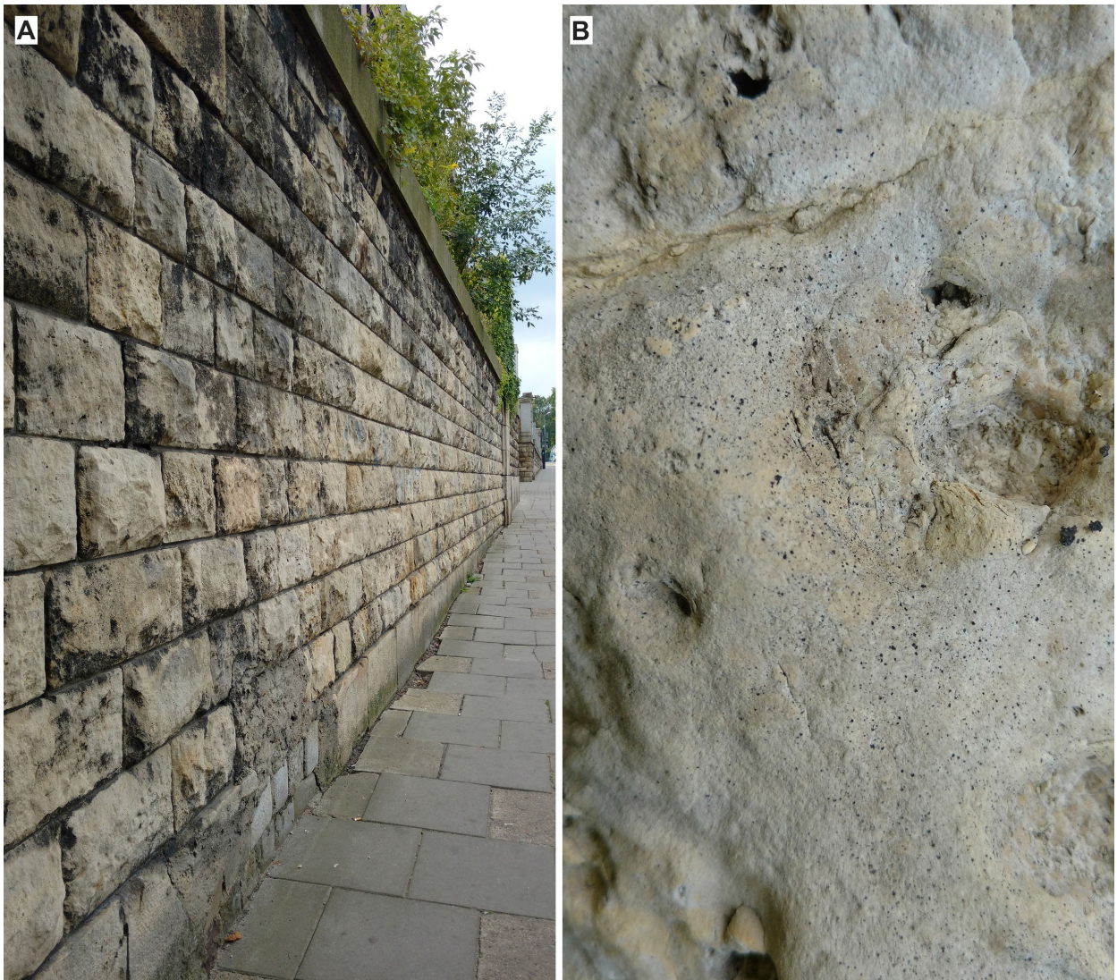
Figure 1. Sampling site. A – view of the dolomitic wall in Kraków; B – black fungi colonization at the surface and in pits of a dolomite slate.
